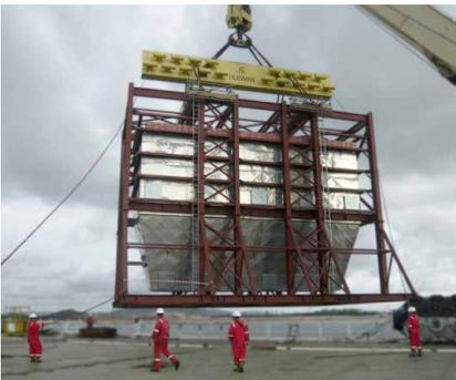
Loading coal mill baghouse with 180 tons and 14-meter height at Batam Anchorage ex barge to *MV Jumbo Javelin*
