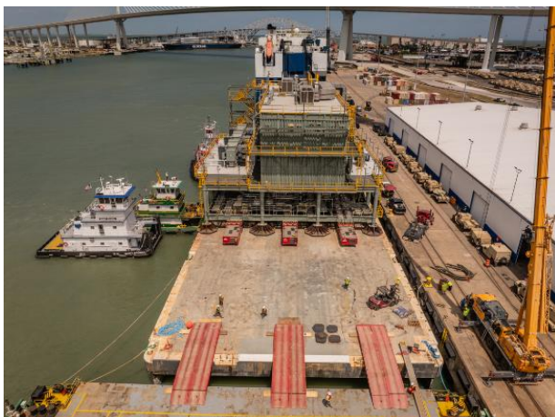
CAPTION: Transfer of the over 25,778 CBM module from the barge to the deck carrier at the Port of Corpus Christi, Texas, USA
