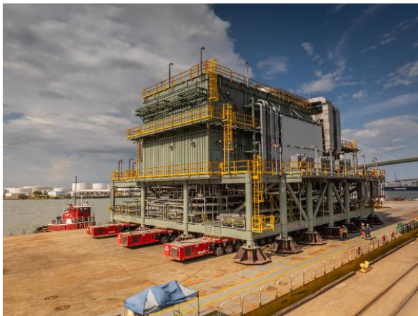
CAPTION: Preparations for the transfer of the over 25,778 CBM module from the barge to the deck carrier
