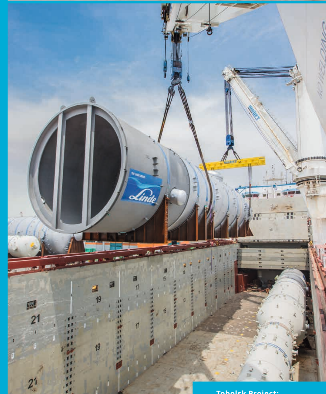
Tobolsk Project: C3 Splitter lifted in Ulsan Port, Korea
