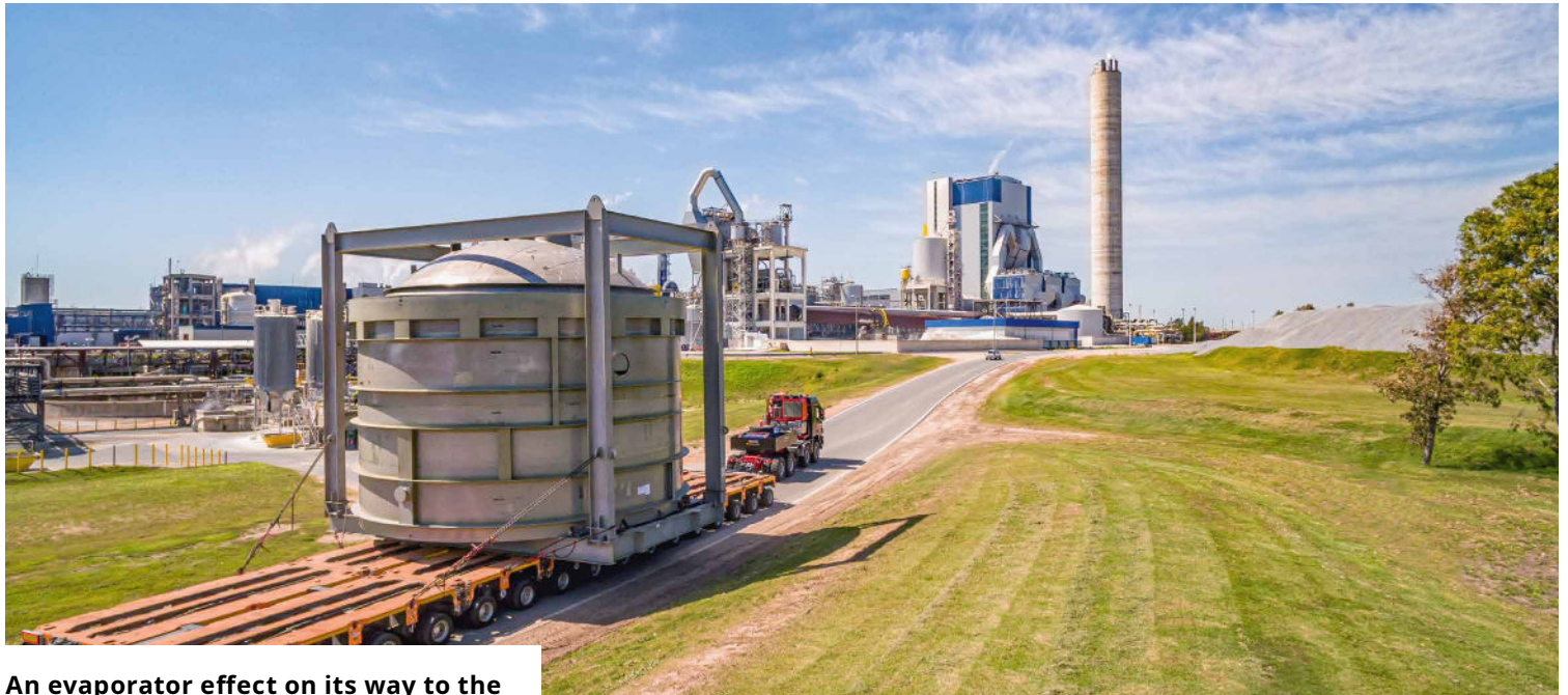
An evaporator effect on its way to the storage area at UPM Fray Bentos
