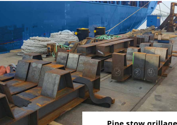
Pipe stow grillage ready for installation on board
