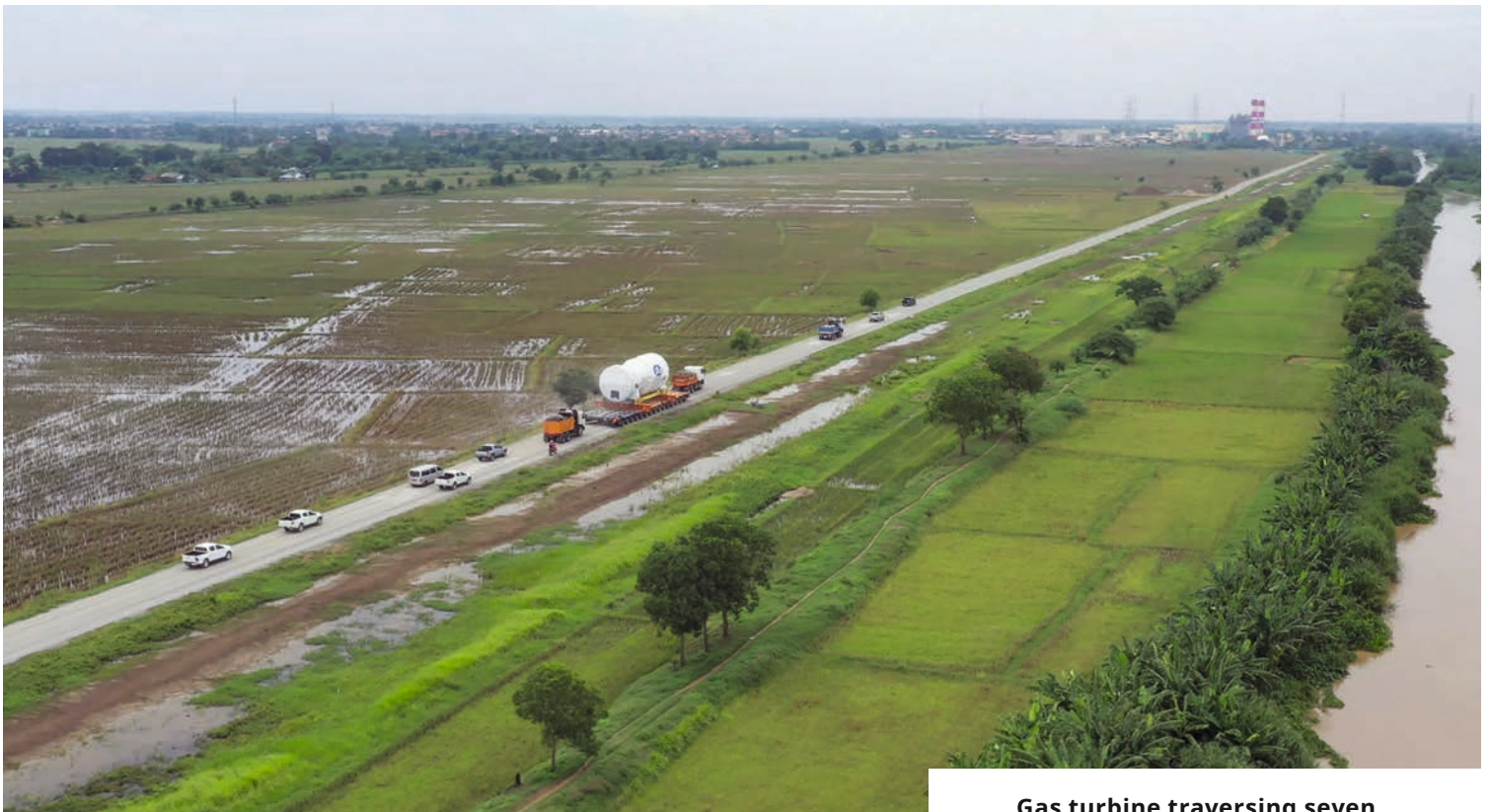
Gas turbine traversing seven kilometers on the purpose-built roadway to the construction site
