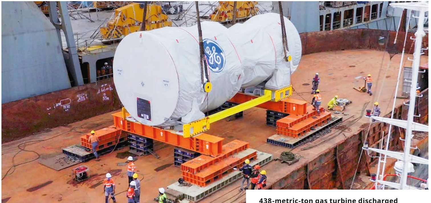
438-metric-ton gas turbine discharged directly from the vessel to the barge at the Port of Tanjung Priok
