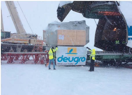
Positioning the transformer on the loading ramp in Helsinki
