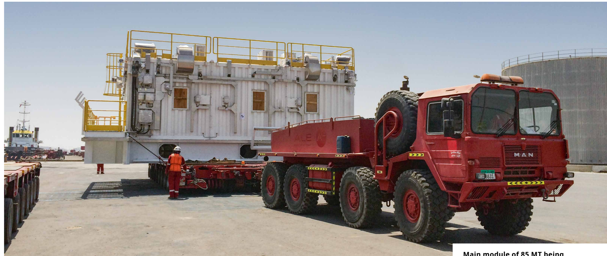
Main module of 85 MT being shifted alongside the berth
