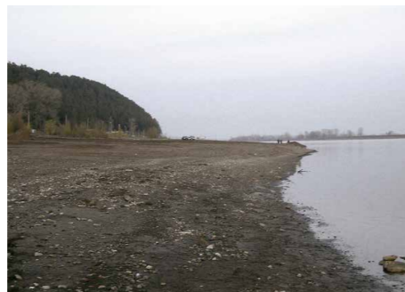
Start of jetty construction
