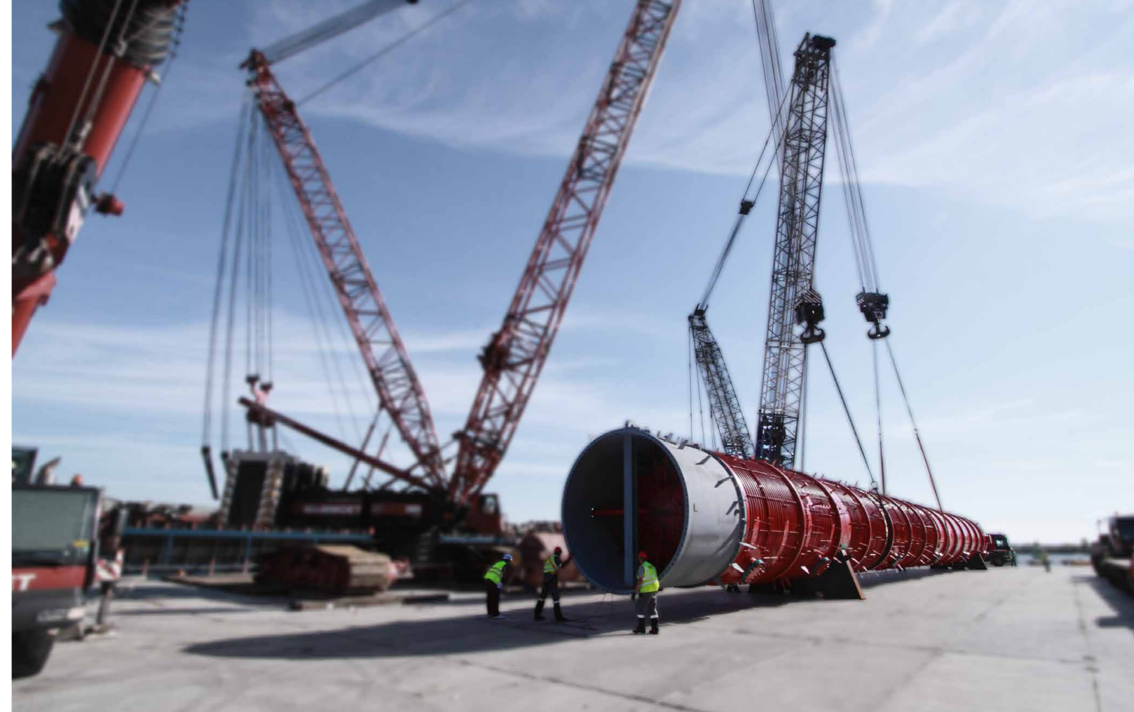
Lifting operation at jetty
