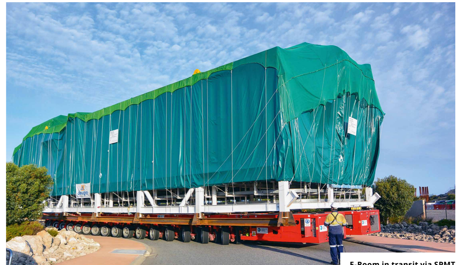
E-Room in transit via SPMT from Henderson wharf to client's storage yard
