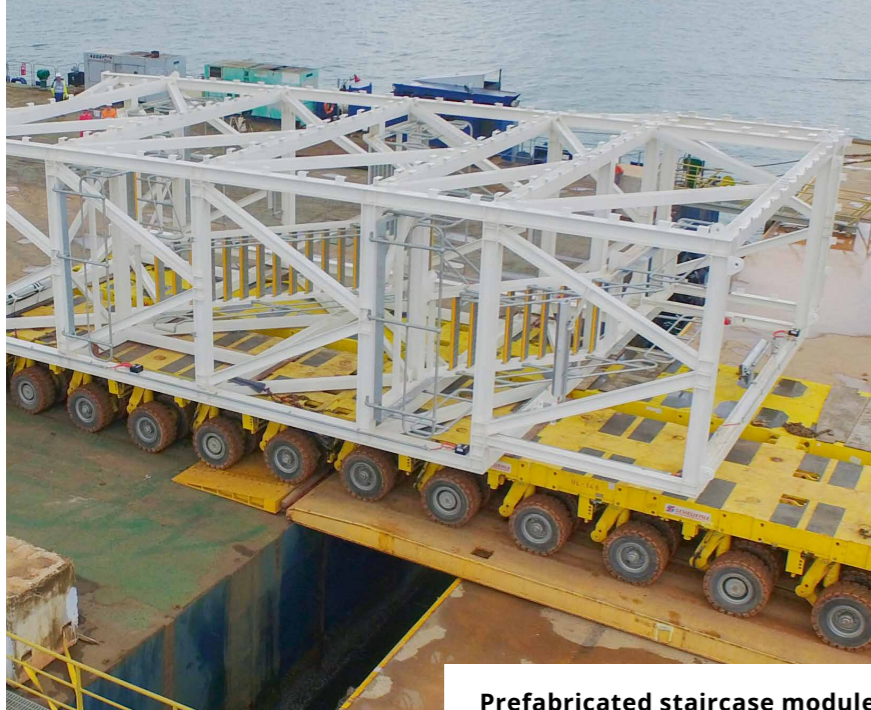
Prefabricated staircase module being rolled onto vessel
