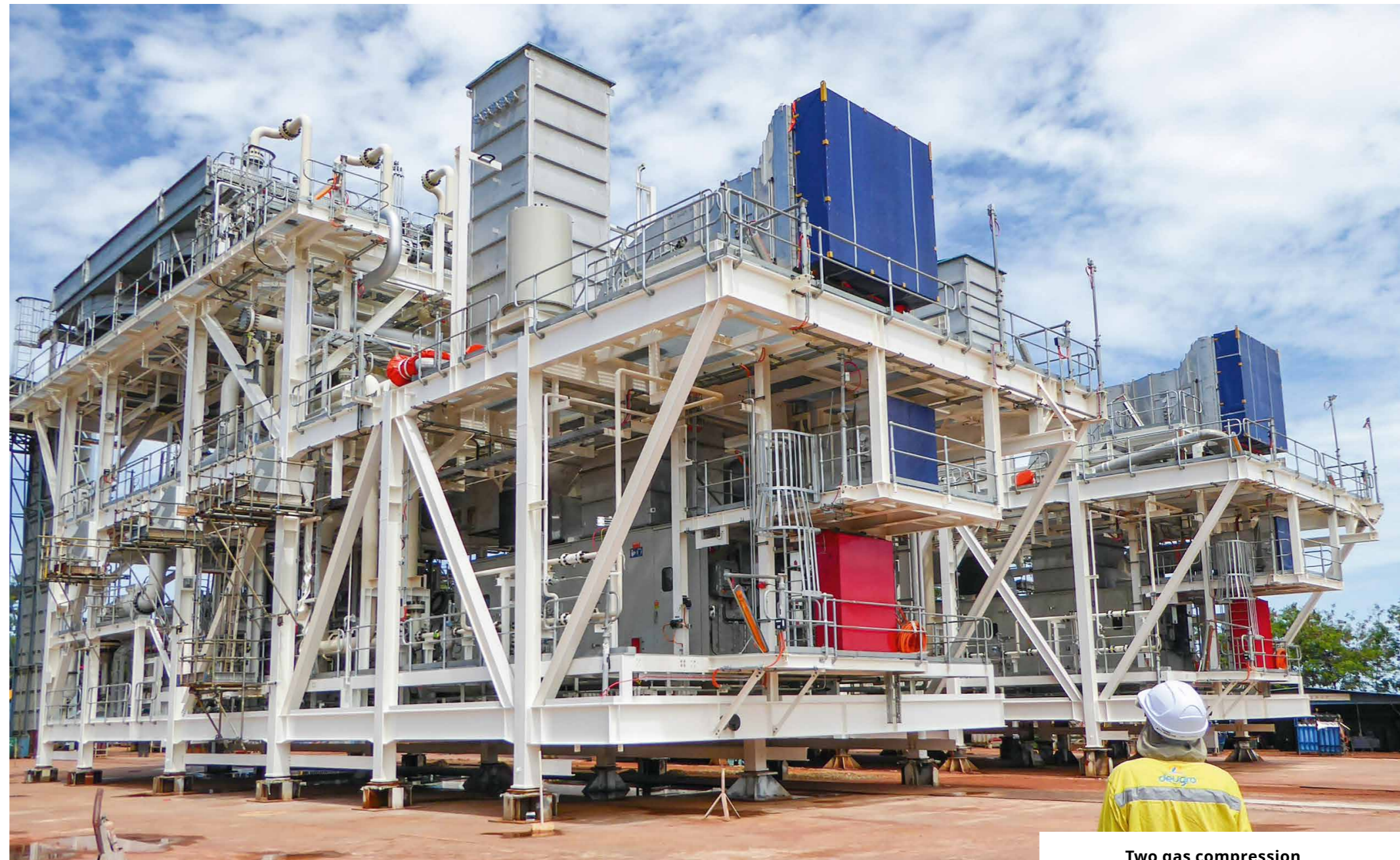
Two gas compression modules awaiting loading at Sekupang, Batam, Indonesia
