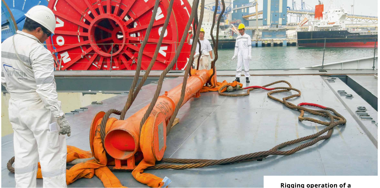
Rigging operation of a spreader beam on board the MV Palabora
