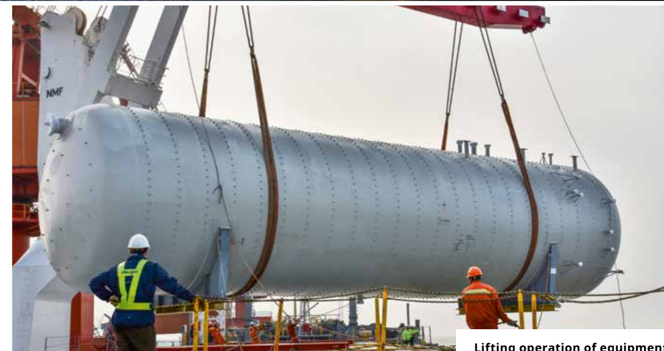
Lifting operation of equipment for the Tobolsk Project
